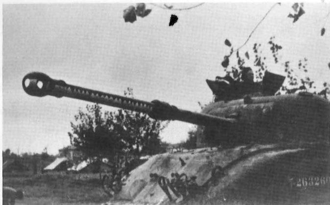
A rare view of a Sherman IC (Hybrid) Firefly with cast-hull front. This view also shows nicely the fake muzzle brake located half-way down the barrel and the disruptive camouflage scheme used to disguise the tank's tell-tale longer barrel. [PA-115712]
